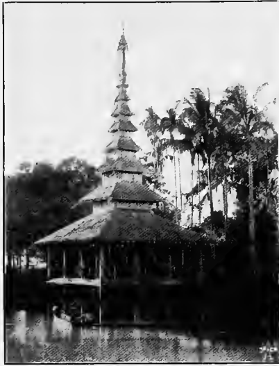
5. LANDING-STAGE IN THE TIDAL REGION.
